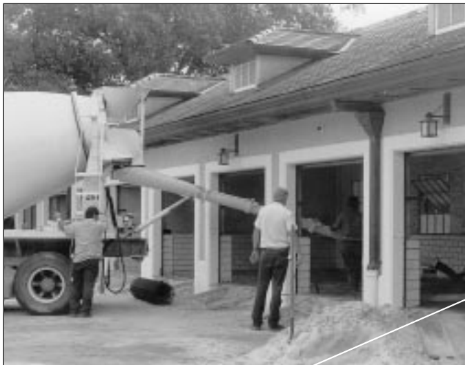
Above: Pouring concrete to bring the new floor 15 inches above grade.
