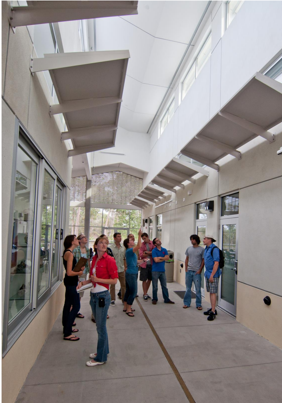
Photo 1: Light gathered from clerestory windows high up is reflected from light shelves into interior rooms. Photo by Archbold Biological Station.
