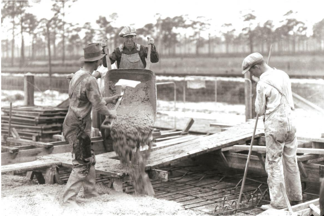
Photo 3: Workers pour foundation for the storehouse, 1930. Photo by Alexander Blair.
